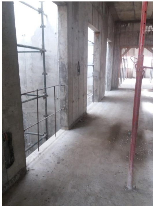
Figure 14: Fabricated steel rods used as barriers around floor holes to protect workers from falling
