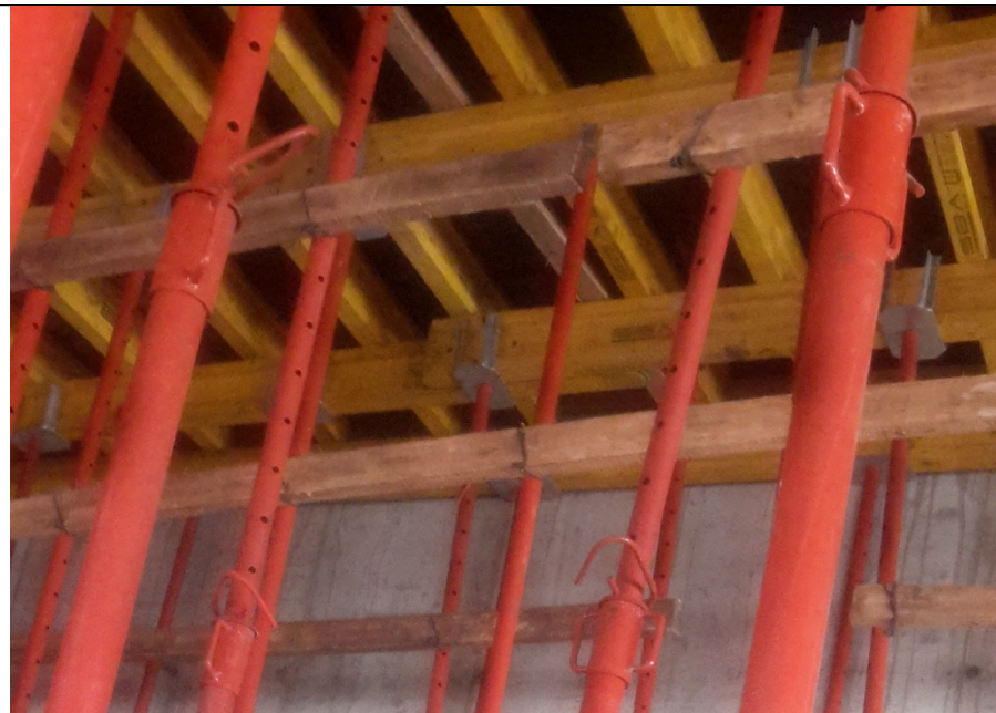
Figure 3-4: Props with Clearly Defined Handle of Adjustment
