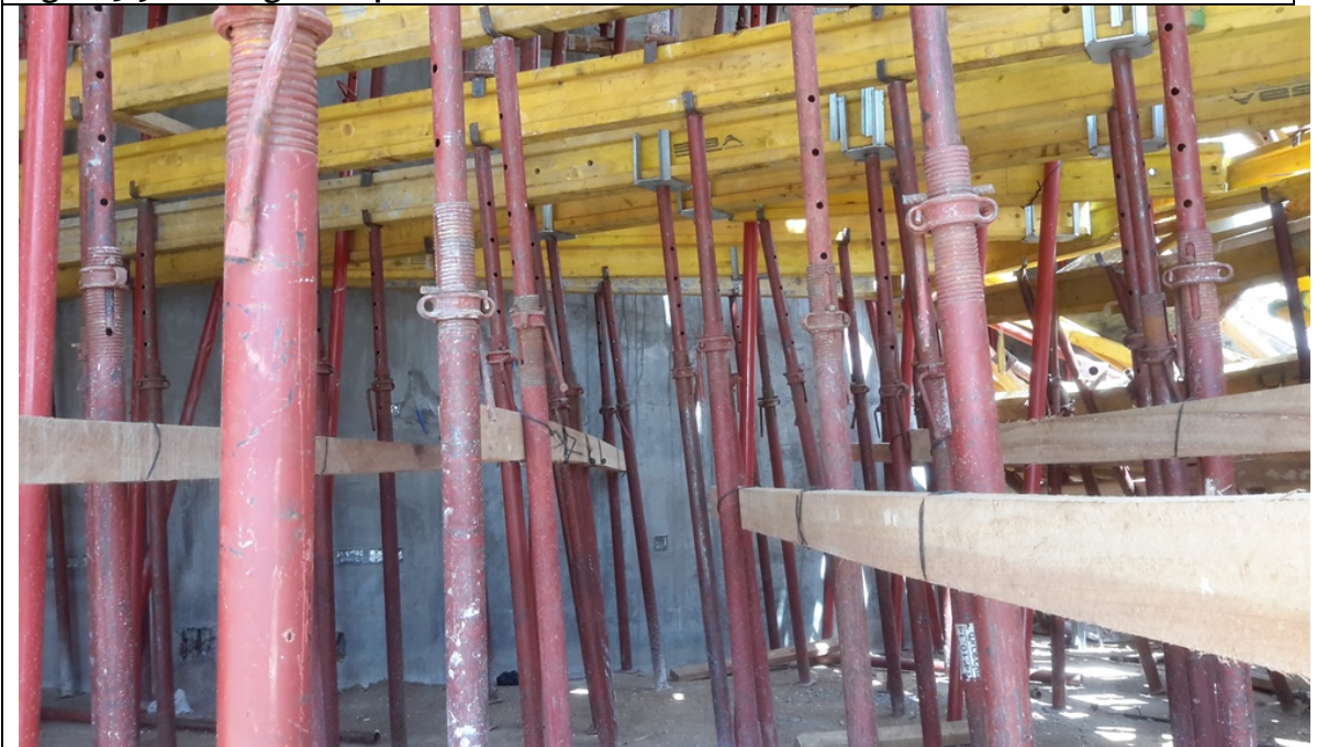
Figure 3-9: 'Bracing of Props – Another view
