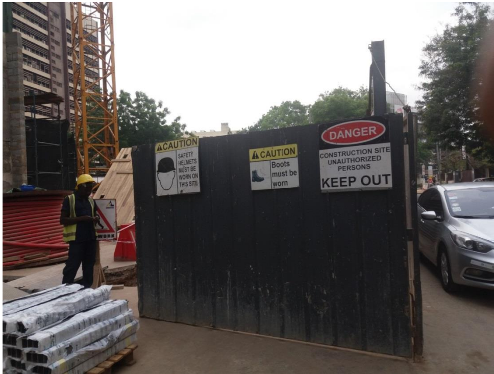
Figure 21: Signages posted on the entrance gate to remind workers to wear their personal protective equipment always on site.
