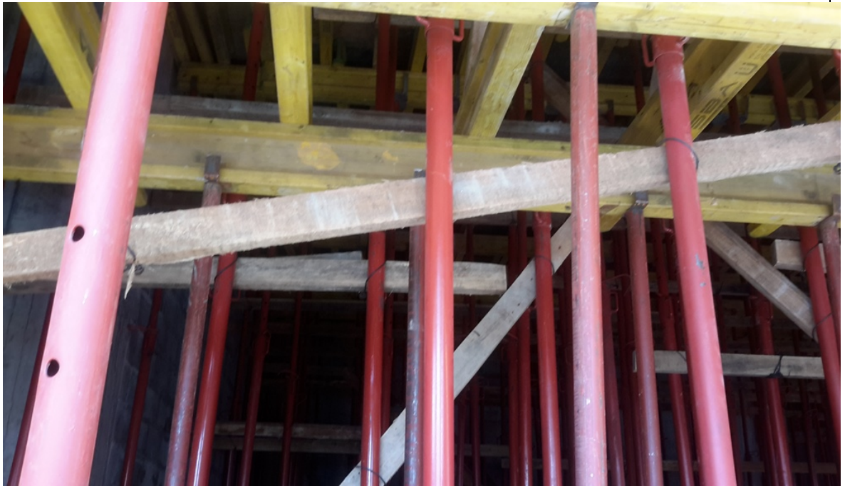
Figure 3-9: 'Bracing of Props – Another view
