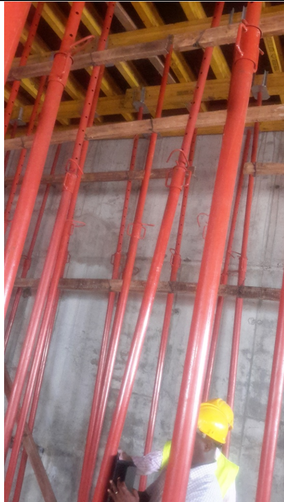
Figure 3-4: Props with Clearly Defined Handle of Adjustment
