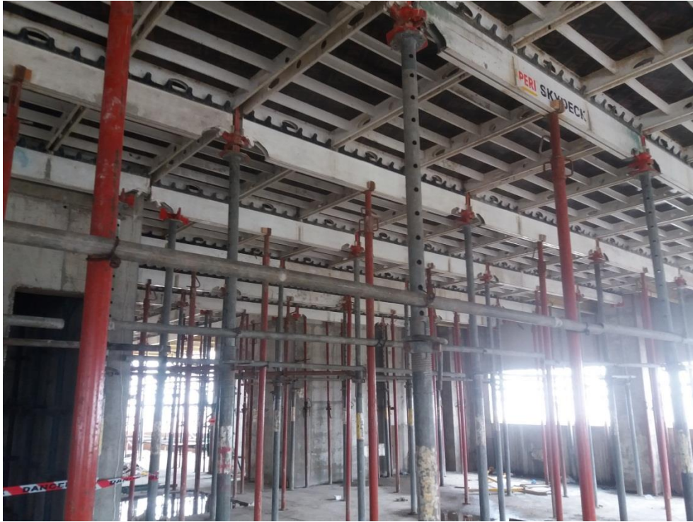
Figure 17: Slab formwork adequately supported by solid steel props.
