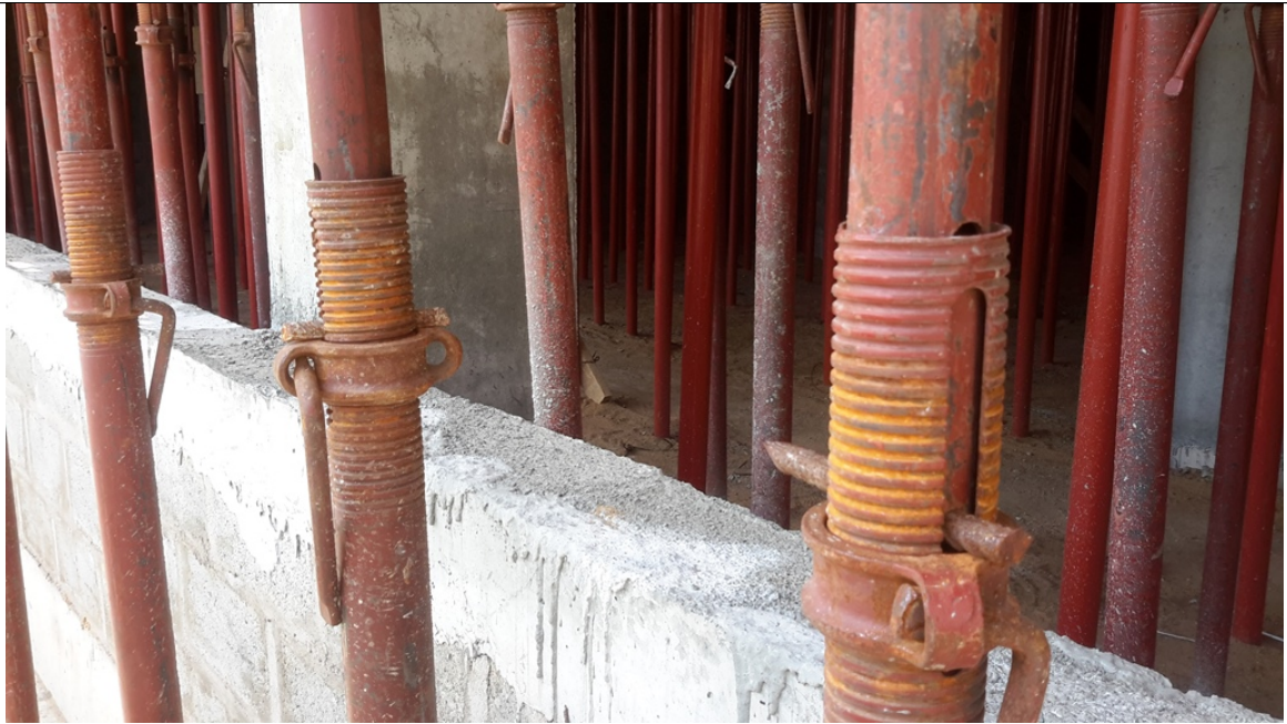
Figure 3-5: Different type of Pin of Fixation
