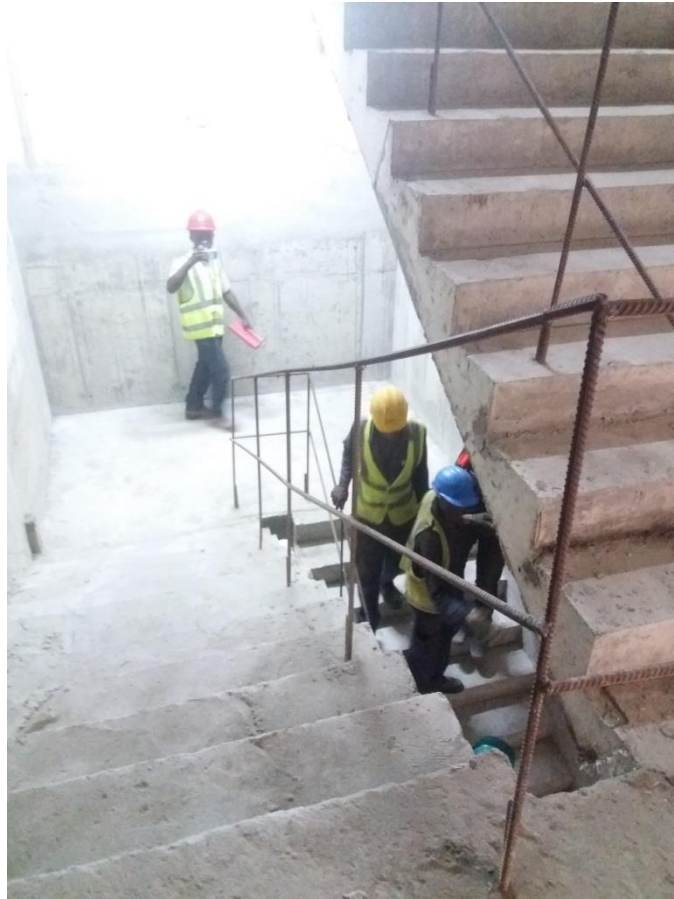
Figure 15: Fabricated steel rods used as handrail and barrier for the staircase to protect workers from falling
