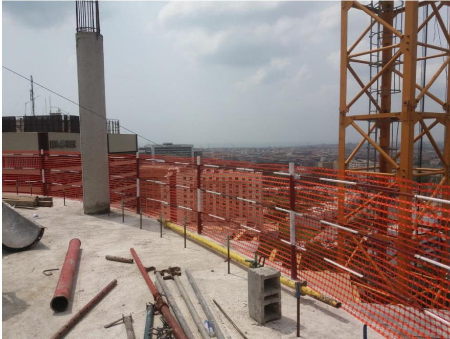
Figure 13: Fabricated steel rods painted red and white, used as barriers on the edge of the floor slab with red net around them to protect workers from falling
