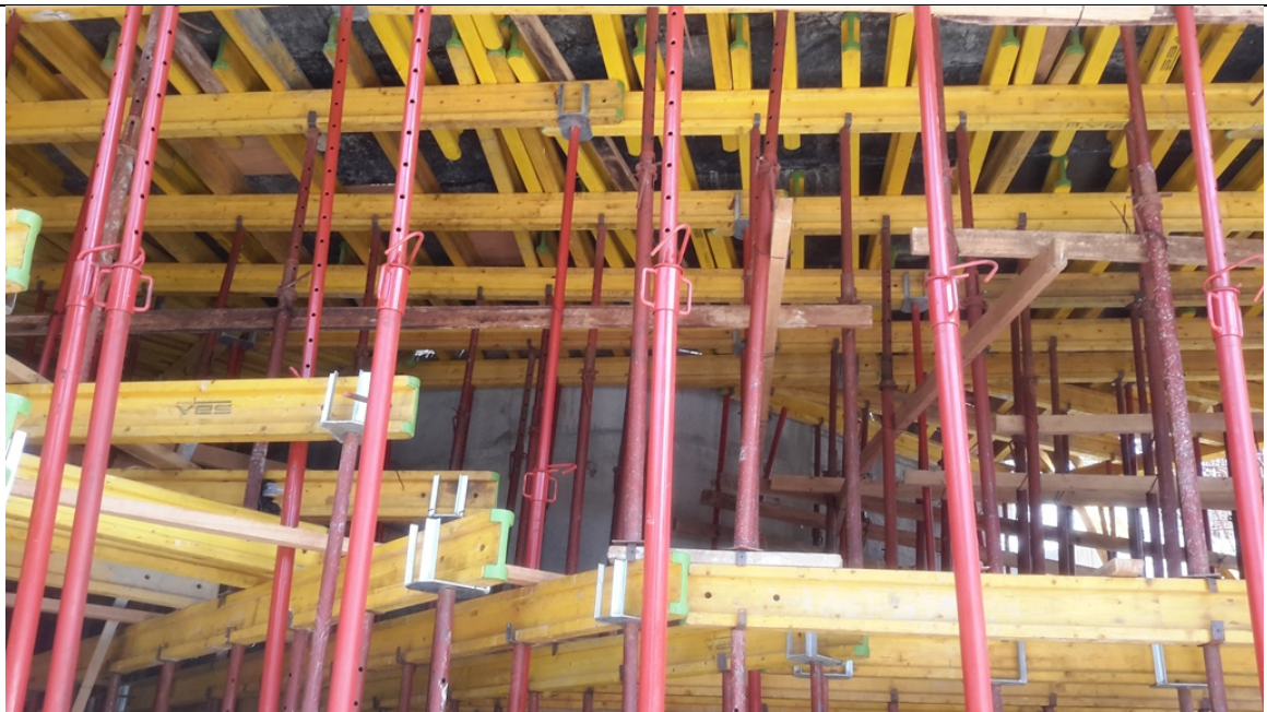
Figure 3-6: Props supported off Joists
