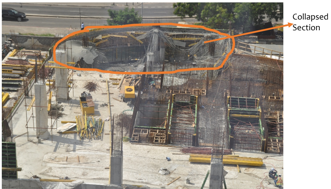
Figure 1-1: View of Work to date
