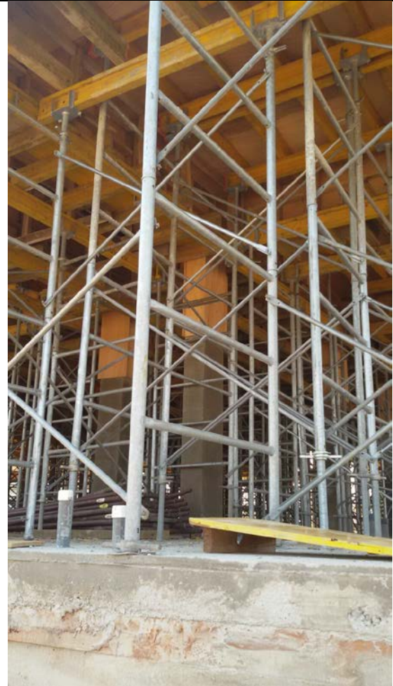
Figure 3-4: Props with Clearly Defined Handle of Adjustment
