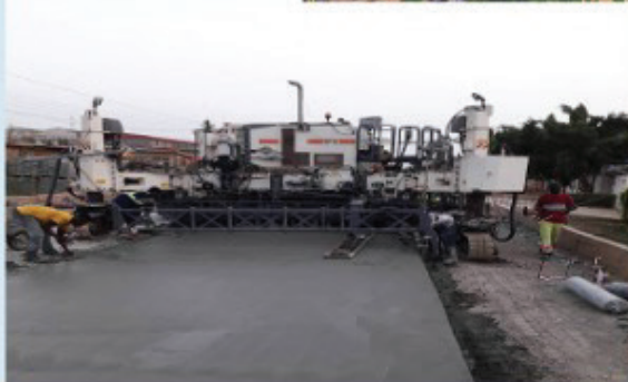
Concrete Pavement for Tema Steel Works Road
